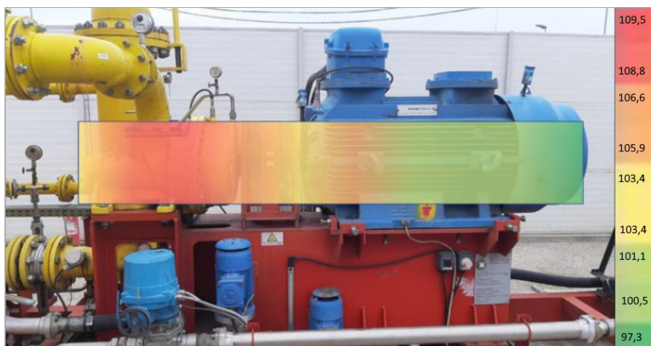
Fig. 2.5 Noise Analysis - Acoustic field distribution - The author's maintenance activities at the studied compressor location - Measured values in dB (decibels). Measurements revealed that the area with the highest acoustic radiation was the compressor housing
